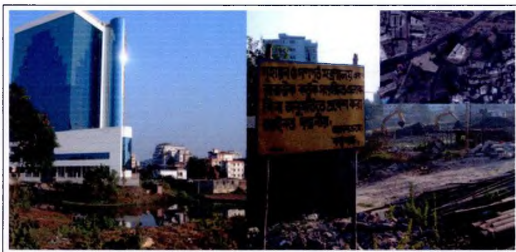
Figure 4.11: Retention area encroached by BGMEA and government authority
