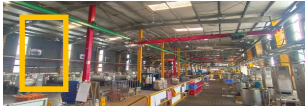
Figure 12: Transparent Wall Sheets at floor
