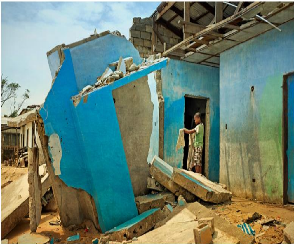
Figure 4.1 (A & B). Image A-(Top) Shoreline of Popo Beach eroded by Coastal Floods. Image B-(Bottom) Six Bedrooms house damage by sea erosion in New Kru Town, Bushrod Island.
