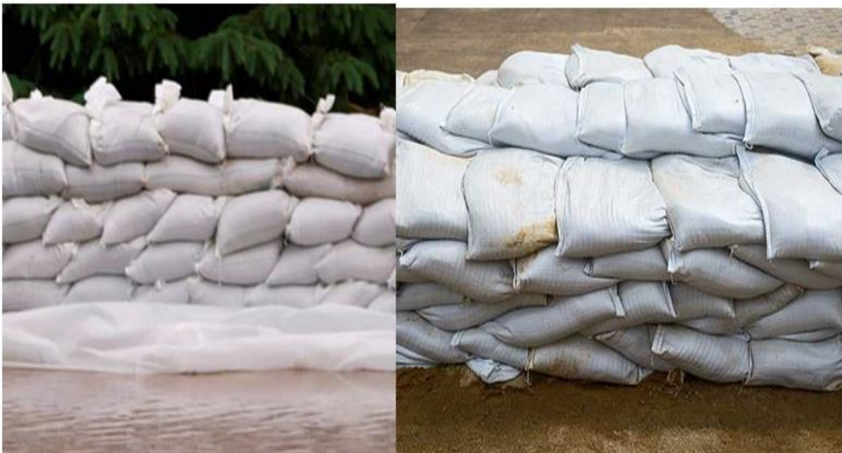
Figure 5.5 (A & B). Images of Sand Berm being used as Flood Wall.
