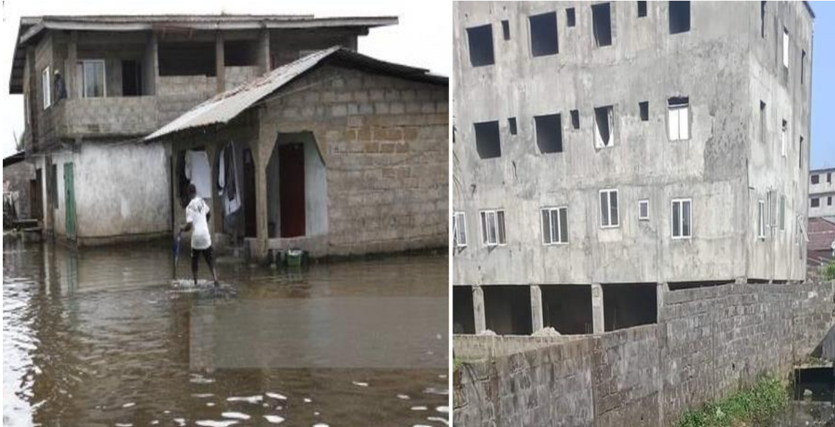
Figure 5.3 (A & B). Images of Buildings elevated above floodwater height via Structural Elevation Techniques in Logan Town and SKD Community on Bushrod Island.
