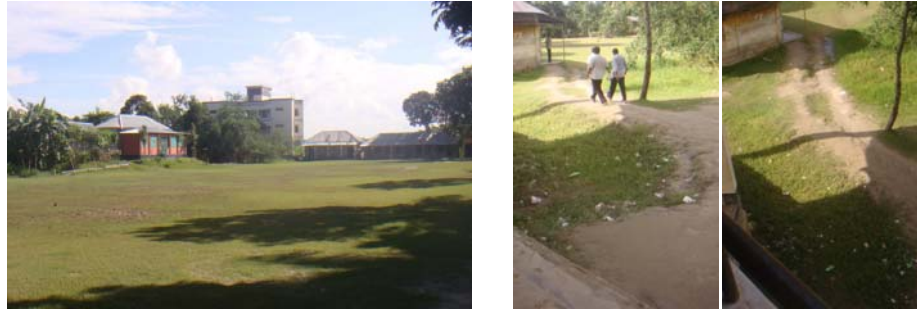
Photo 5.2: Saadipur High School cum Flood Shelter, Sadarpur, Faridpur. There is no designated access path to the shelter
