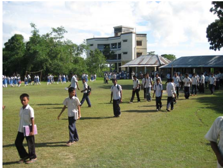
Photo 4.3: Two-storey Saadipur school flood shelter
