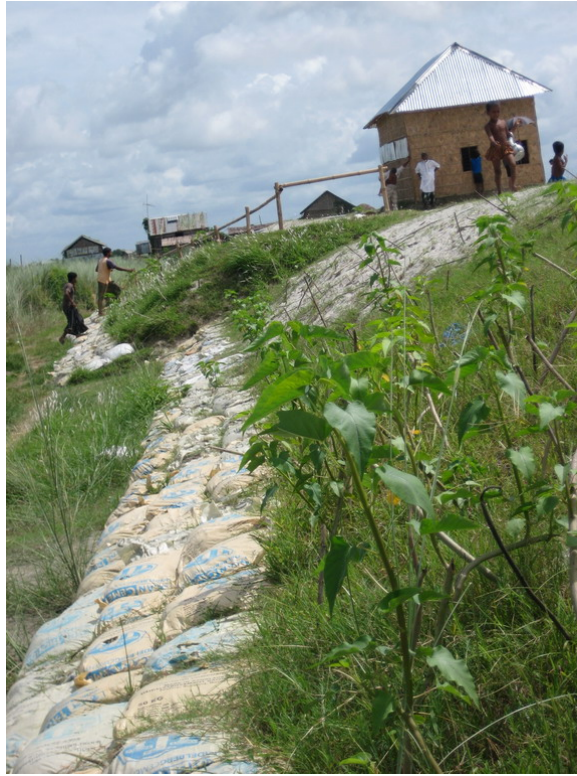
Photo 4.2: Use of geo-bags in protection against wave erosion
