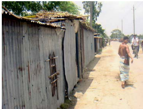
Photo 5.4: Temporary shelter on embankment cum road turned into permanent homes.
