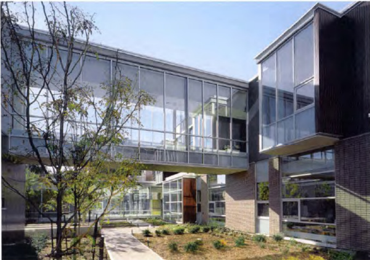
Figure 14: Connection Between Two Buildings
