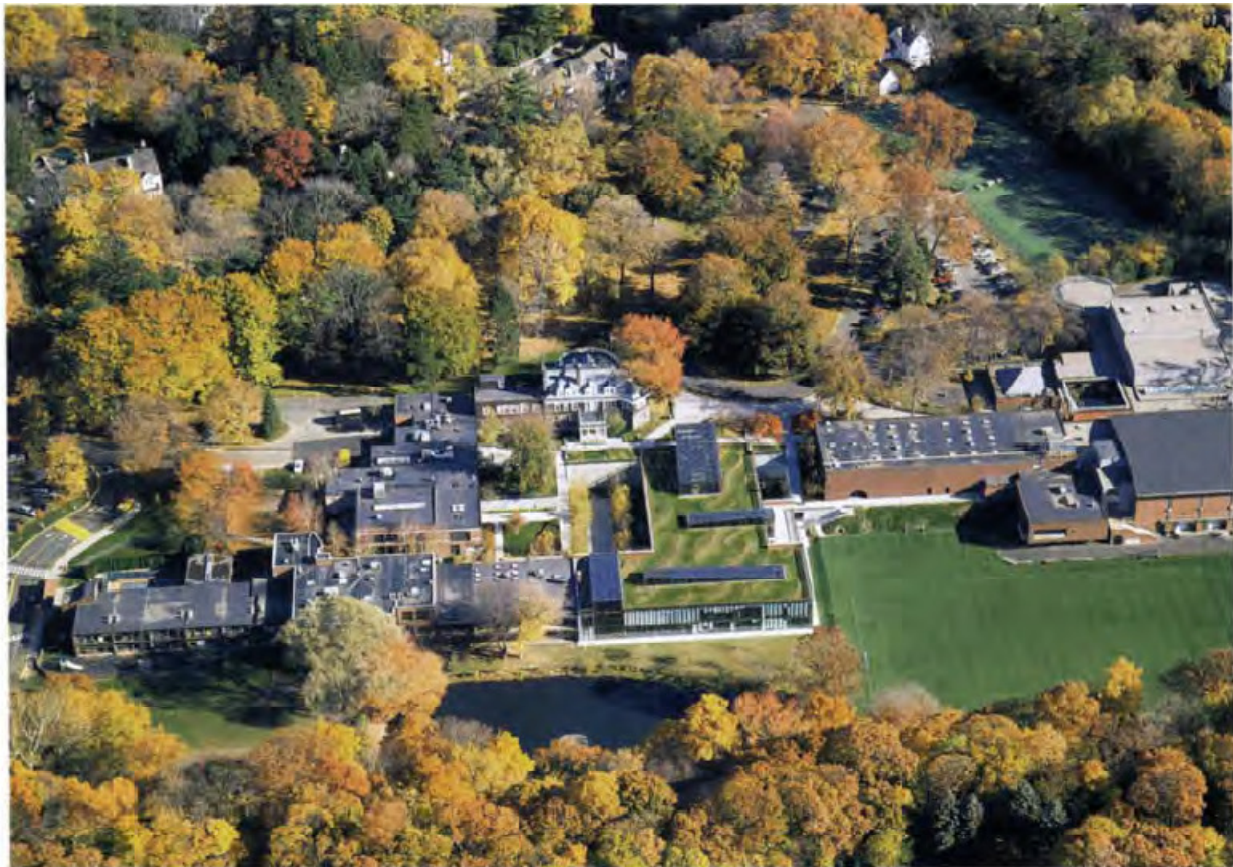
Figure 16: Birds Eye view of the Building
