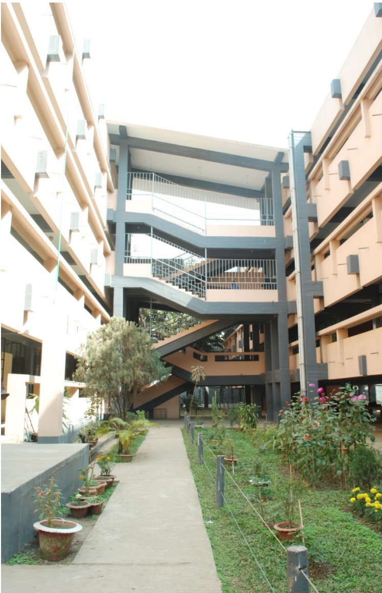
Figure 29: Stairwell at St Joseph High schools
