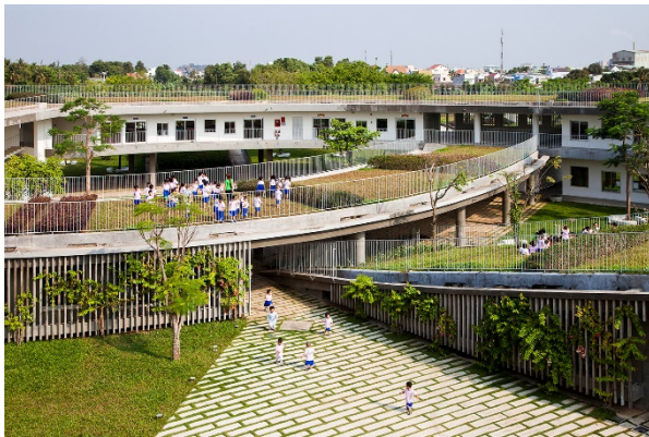
Figure 48: Entry of the school
