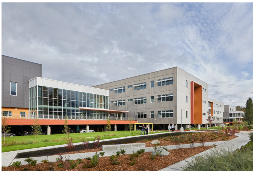
Figure 70: Campus view from street
