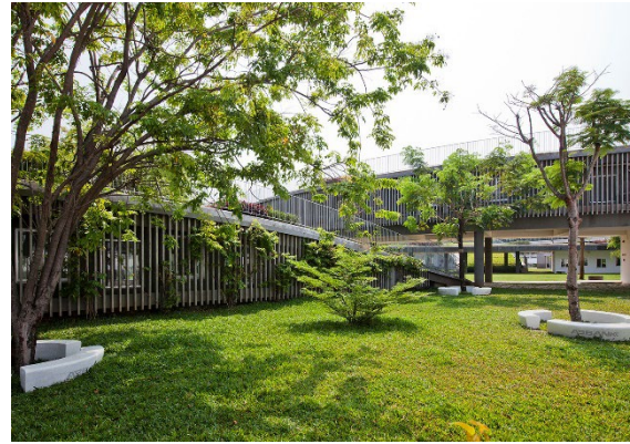
Figure 49: Exterior louvre detail
