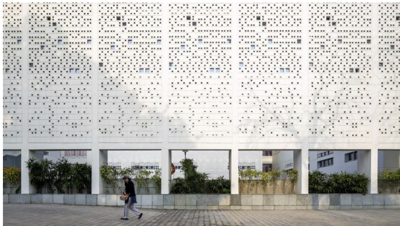
Figure 66: Perforated exterior wall
