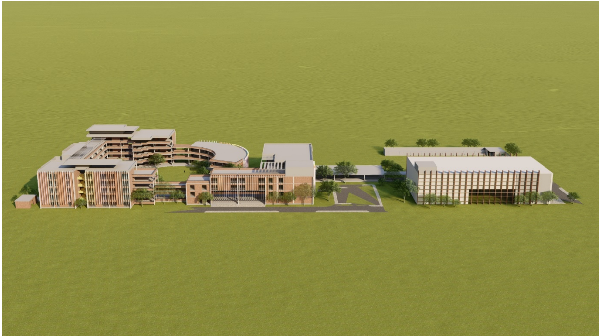
Figure108: View from the west
