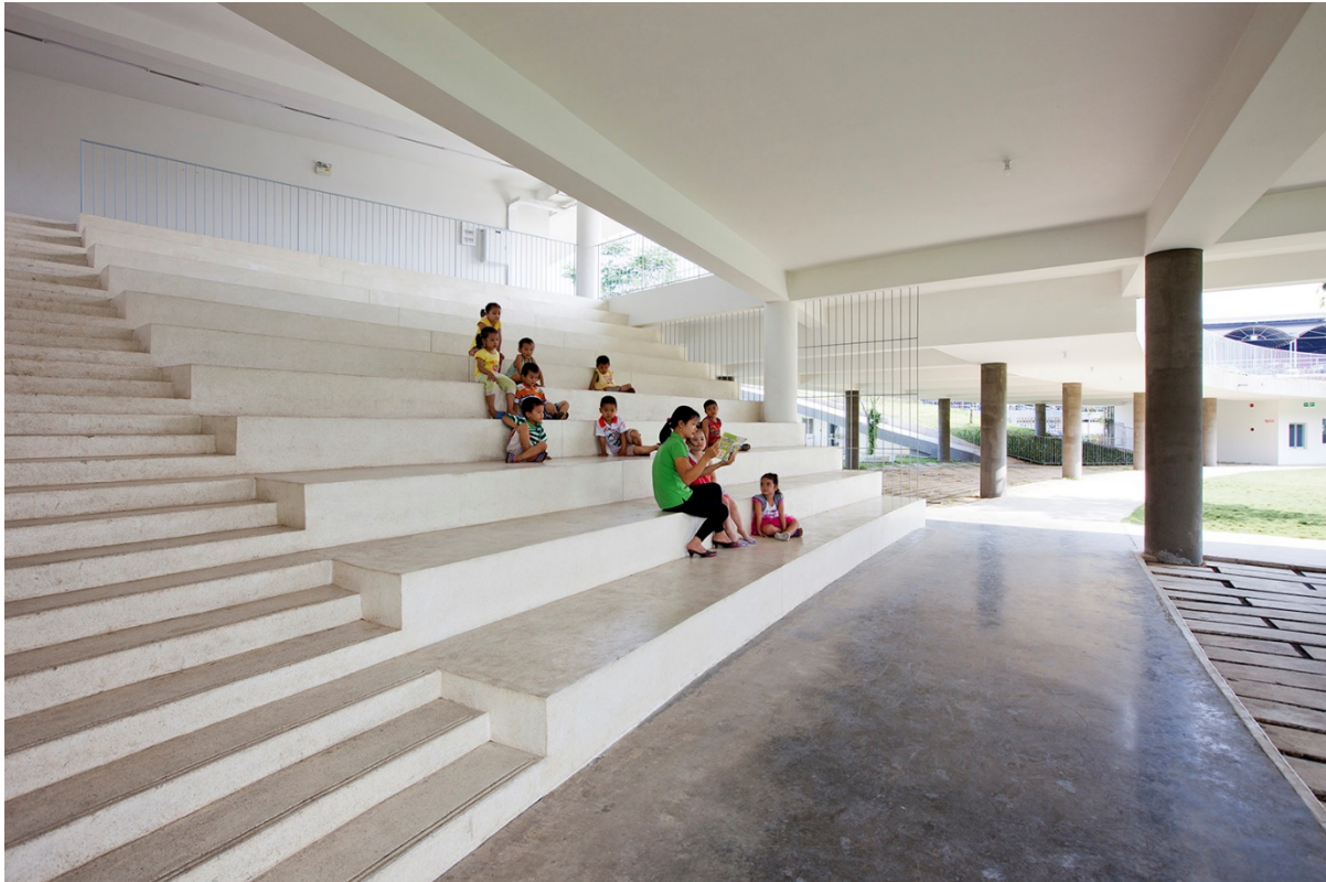
Figure 44: Main staircase & connected corridor
