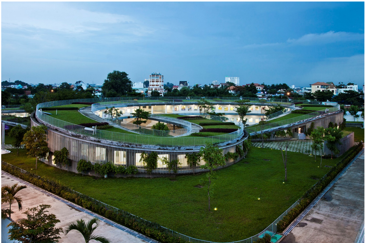
Figure 34: View from south-west side
