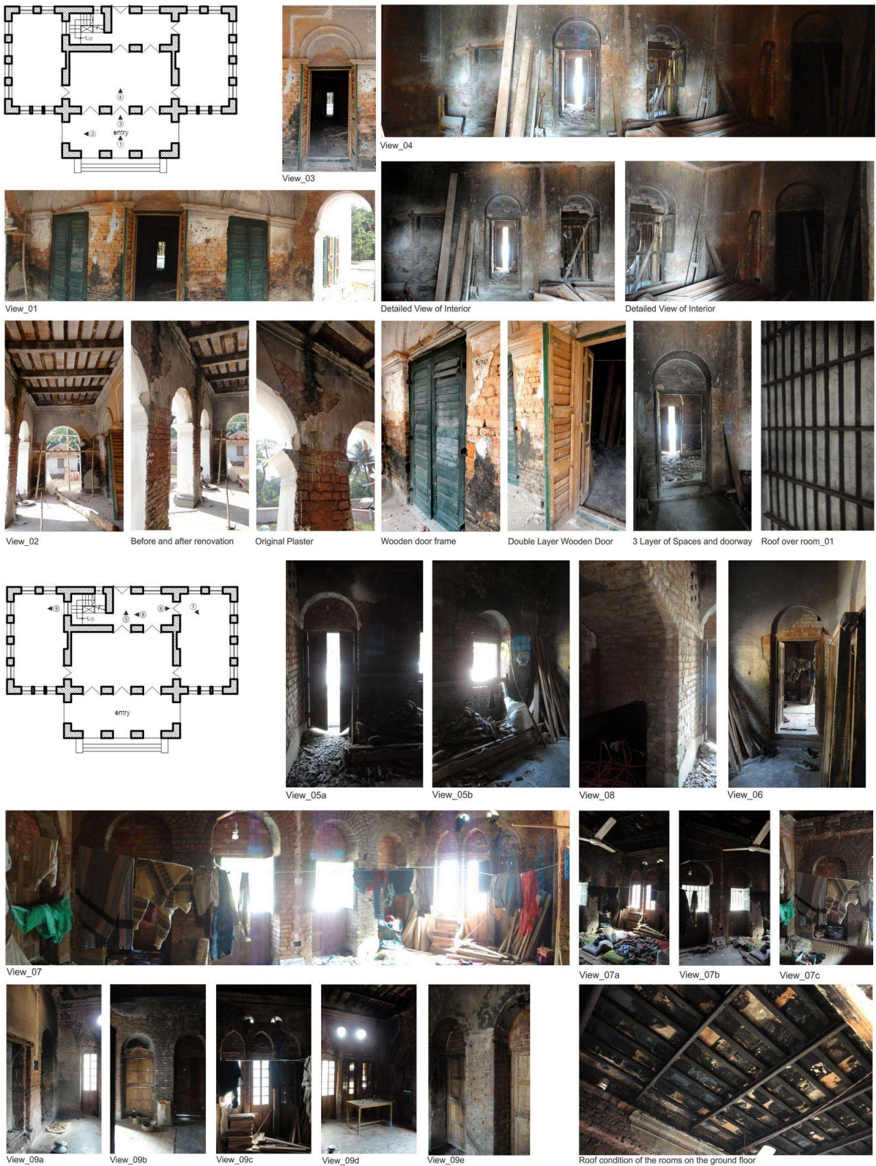
Fig 11:Interior views of the Existing structure Source: Rahman,2012
