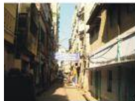
Narrow gaps between buildings and no greenery
