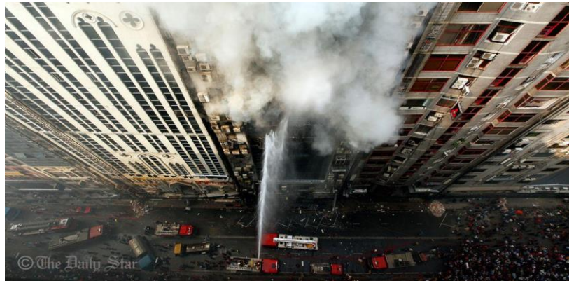
Picture 3: 22-storey building FR Tower fire at Dhaka city.
