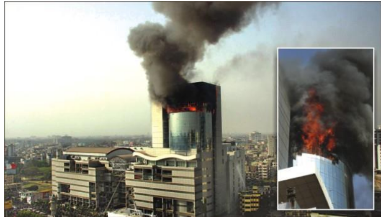
Picture 2: 19 Story building Bashundhara City fire, Dhaka.
