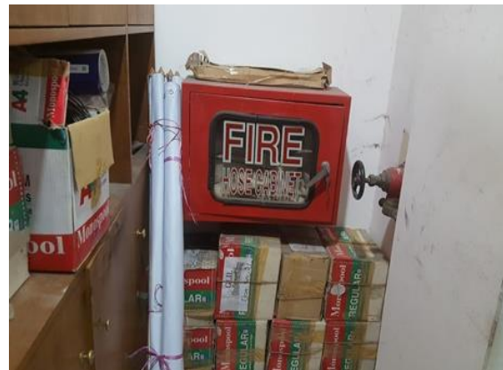
Picture 26: Materials were stored at the riser location
