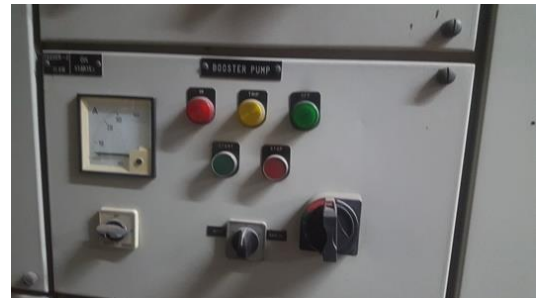
Picture 14: Buster pump control
