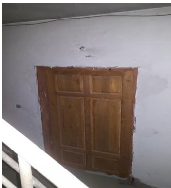
Picture 19: Wooden door at JR Casero
