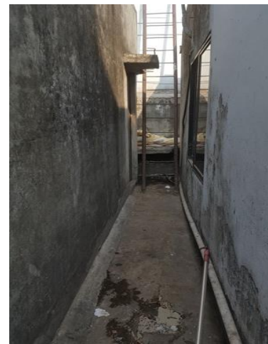
Picture 8: Roof of Siddique Tower is about completely occupied 2 rooms.
