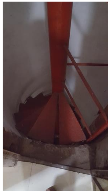
Picture 18: Fire escape at Rupayan Centre
