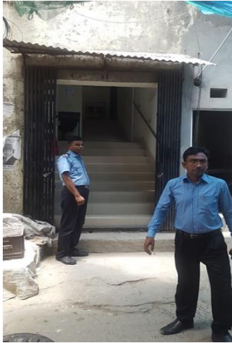
Picture 23: Ambon fire escape directly open outside
