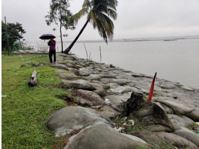
Figure 5.10: Geo bags being used to protect Uria Village from erosion
