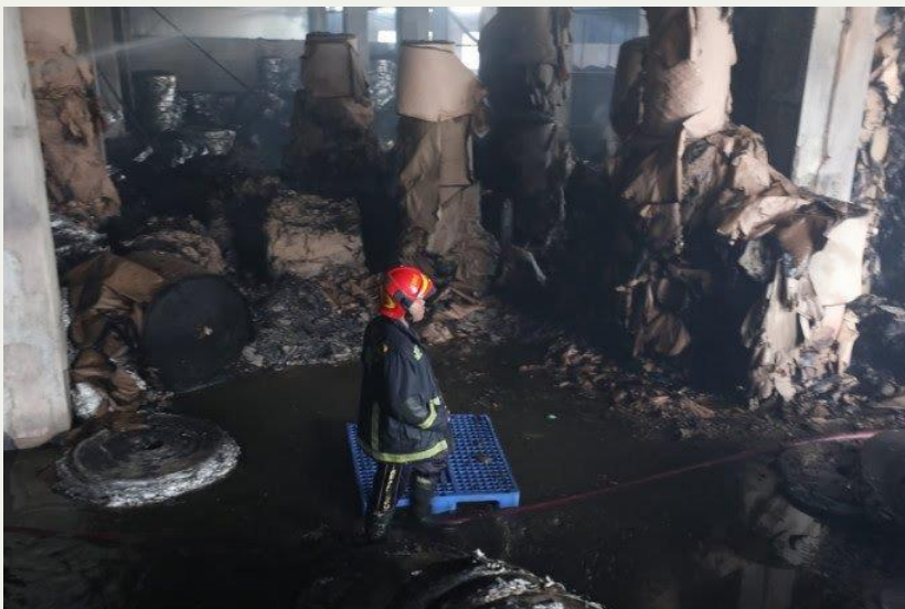
The massive fire that swept through the multi-storey building last Thursday claimed the lives of 53 workers. Photo: Salahuddin Ahmed
