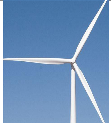
Figure 2.7.3: Three Bladed Horizontal Axis Wind Turbine [15]
