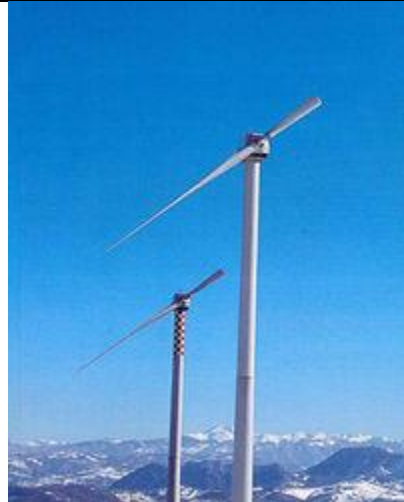
Figure 2.7.1: Single Bladed Horizontal Axis Turbine [15]
