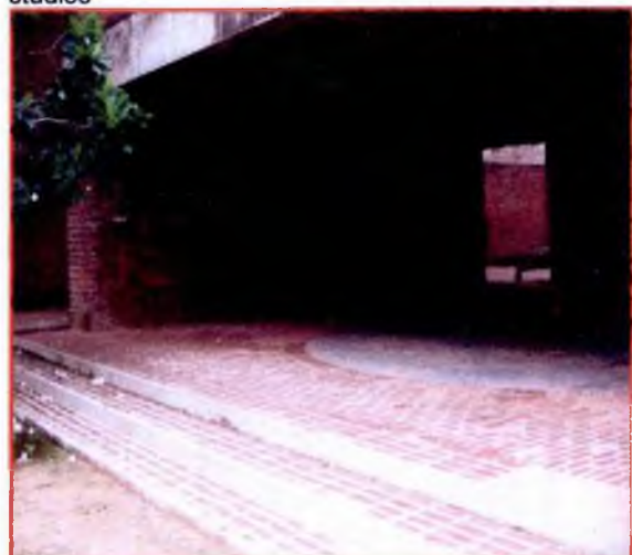
Figure 26: View of the ramp
