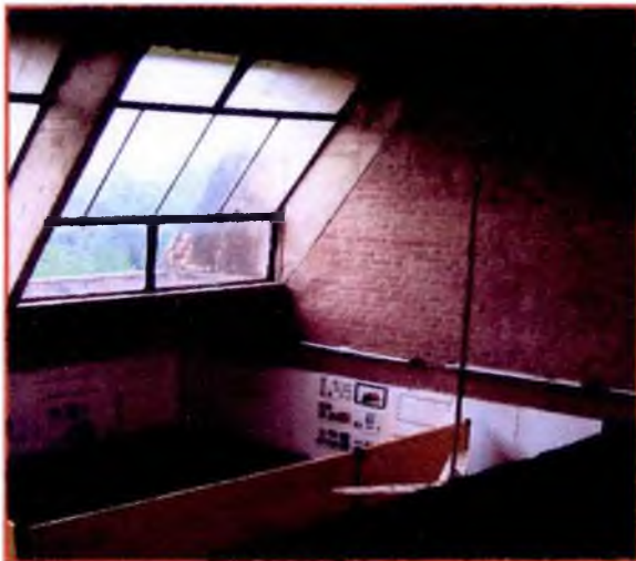
Figure 23: North light in studio
