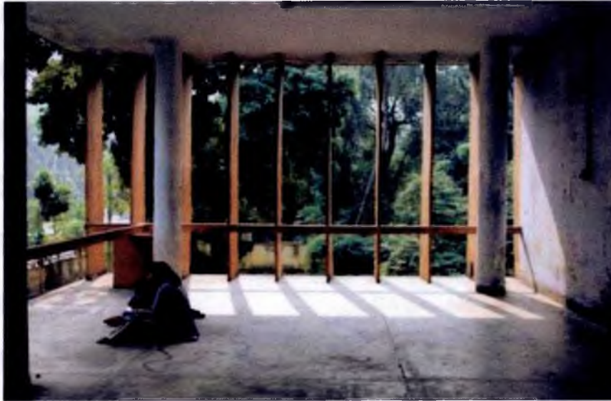
Fig. 5.4. a. Louvers in the south east
