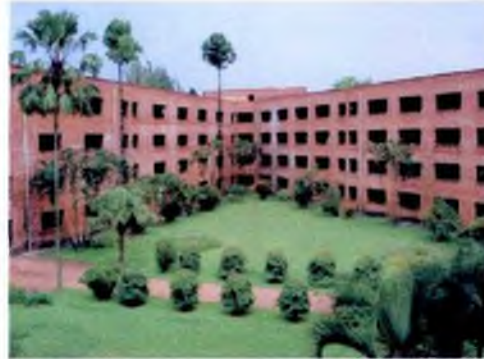
Fig. 2.2.b View of the inside
