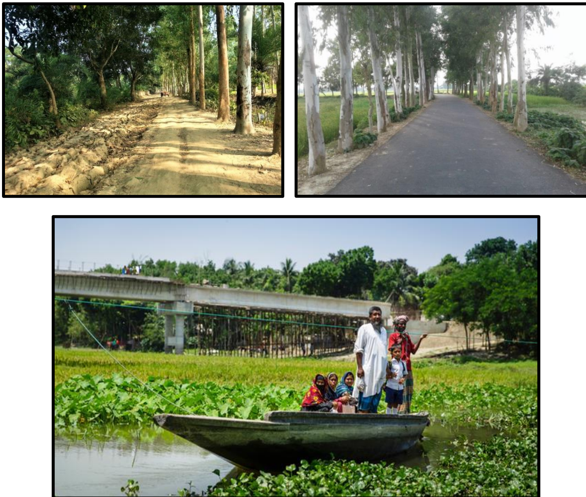
Figure 3.5: Rural road and bridge connectivity
