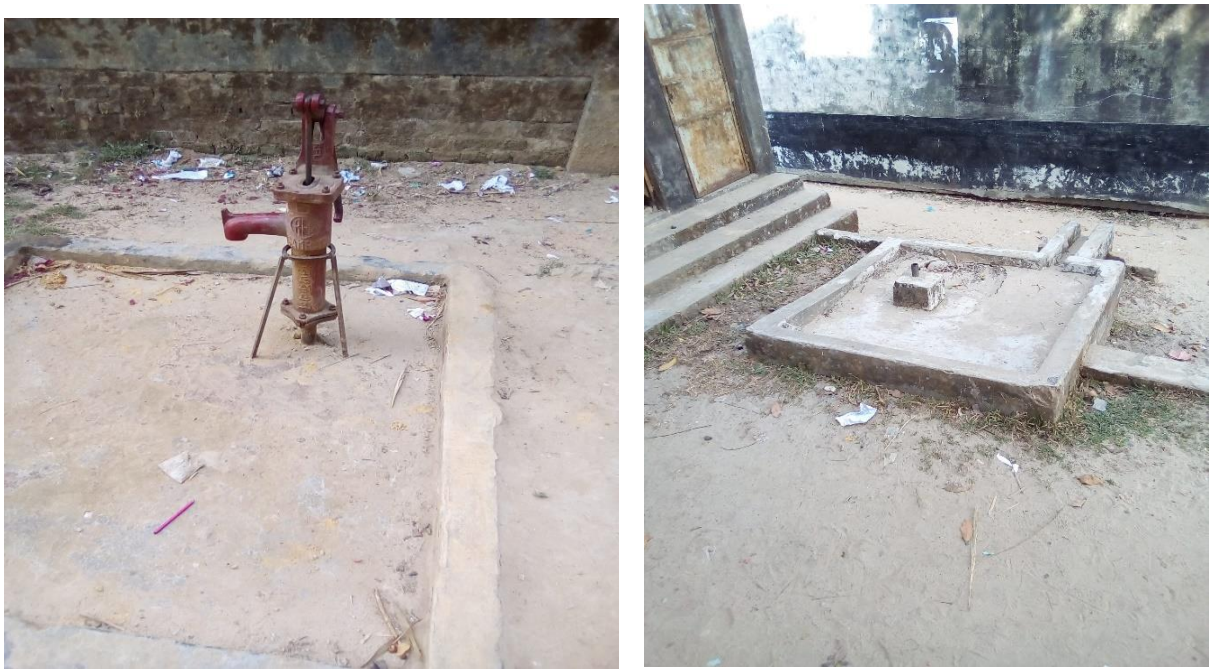
Figure 2: Condition of water supply
