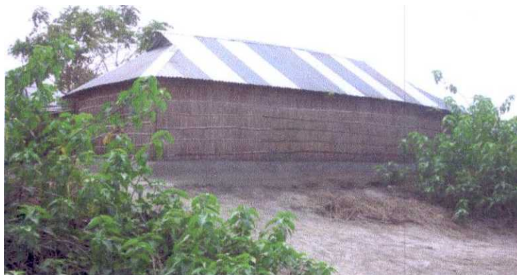
Photo 1 .3: Image of a house made by two different materials (CI sheet and Kaisha)
