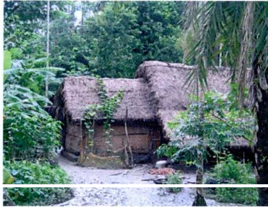
Straw roof and bamboo mat wall
