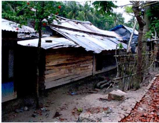
C I sheet roof and wood wall
