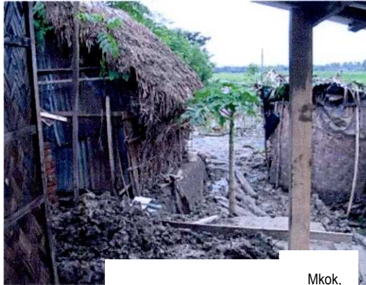
Mkok, Kitchen: straw roof; bamboo frame and straw
