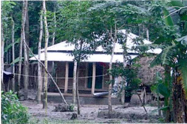
The verandah at the front has four additional wooden pillars.
