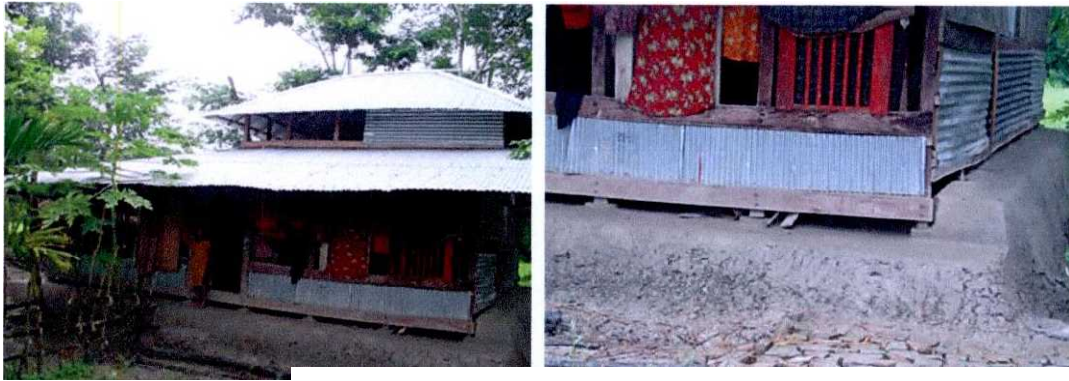
Opening at the front, deep eaves in the roof
