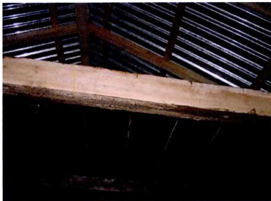
One platform above the head height provides extra space inside the house.
