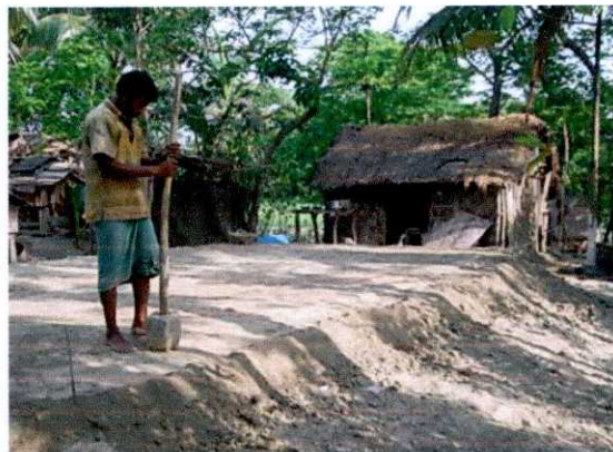
Ramming of earth for preparation of homestead
