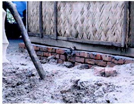
Brick boundary around mud plinth is added later.
