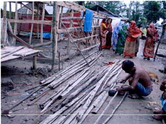
The recipients constructed the houses themselves.
