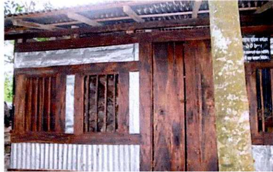
Wood frame is used with C I sheet walls and roof. Wood is used extensively.
