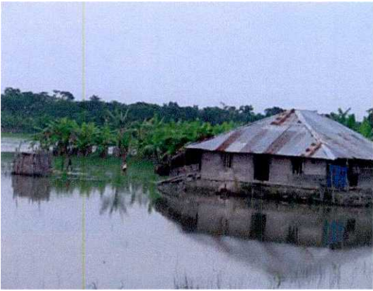
C I sheet roof and wood wal I
