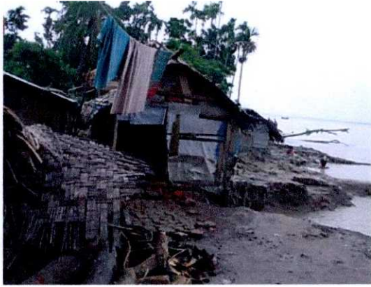
Bamboo mat roof; polythene, wood and bamboo mat wall
