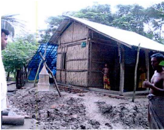
Homestead plinth heightening is done in the later reconstructions.
