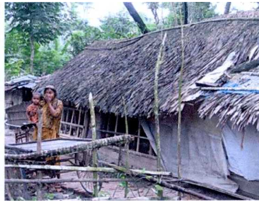
Chicken coop: hogla roof; wood, fishing net and polythene walls; mud plinth.
