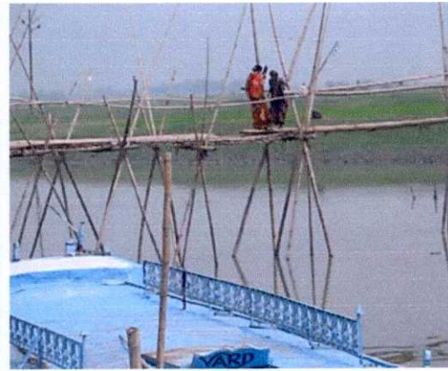
Bridges of bamboo plank and pole are used in many places of the country that can be used here too (source: author)
