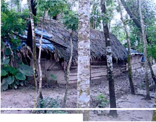
llogla roof and wood wall
