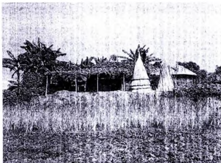
Photograph 1: Homestead raising at char areas
