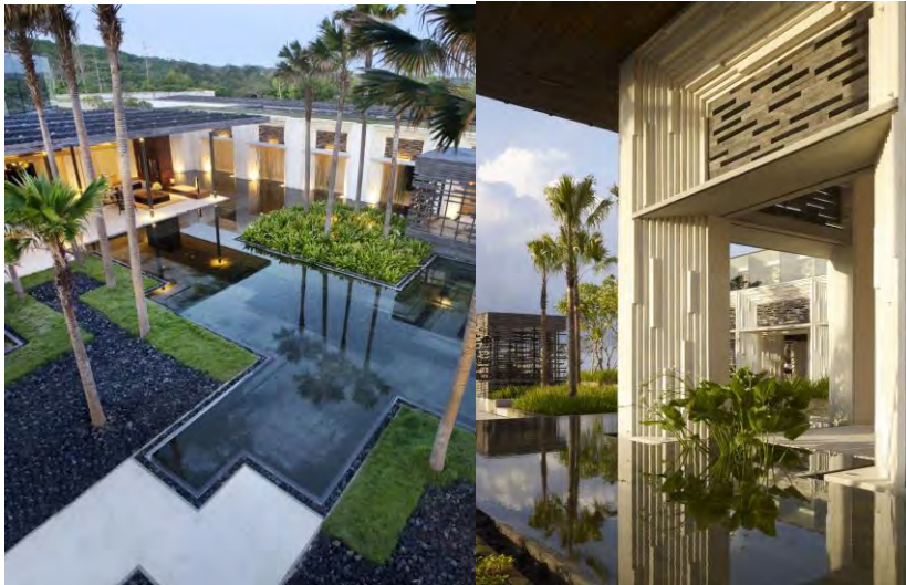
Figure 49,50 and 51 : Views of pool, courtyard and bar Source: www.alilahotels.com , 2018
