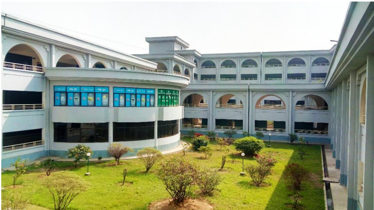
Figure 19: Hajj Camp in Ashkona. Source: Author, 2019
