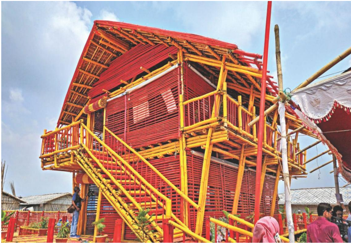
The two-storey eco-friendly learning centre for refugee children at Kutupalong camp in Cox's Bazar. Photo: Star
