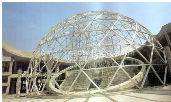
Fig: 5.1.3.Steel Structure of the Planetarium
