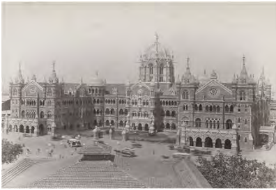
Fig 2.5.3: Bori Bunder Station
