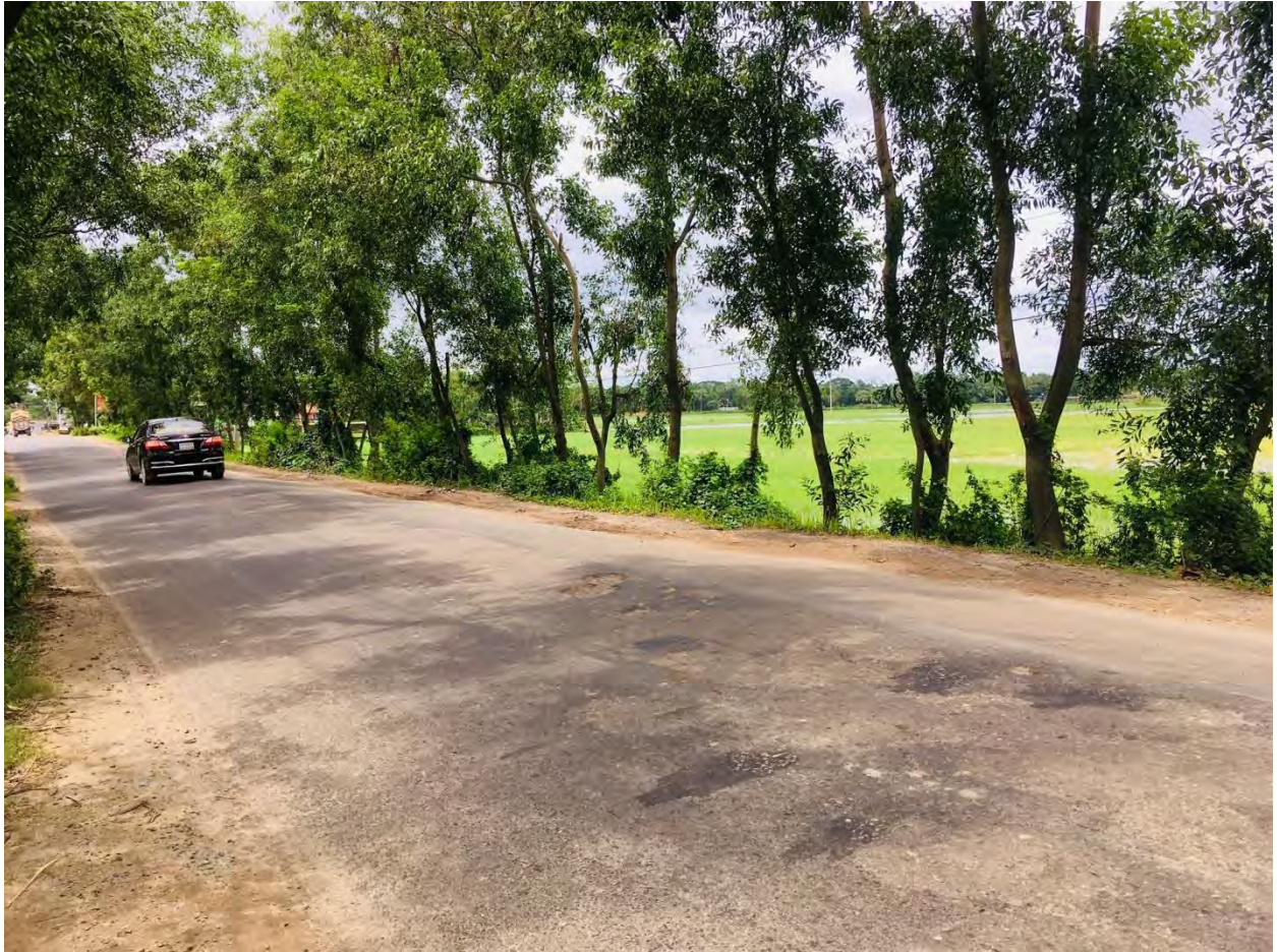
Figure: Site Photography(Source: Author)
