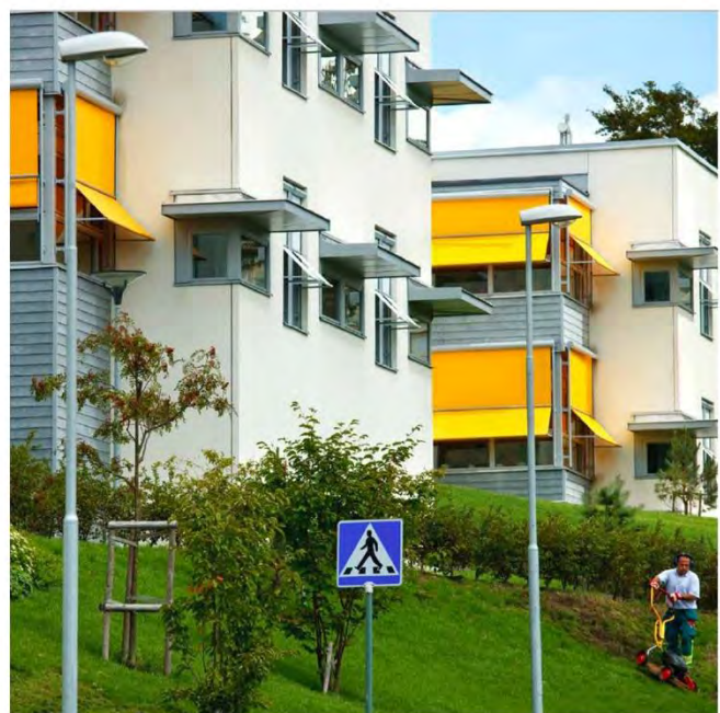
Exterior view of facade
