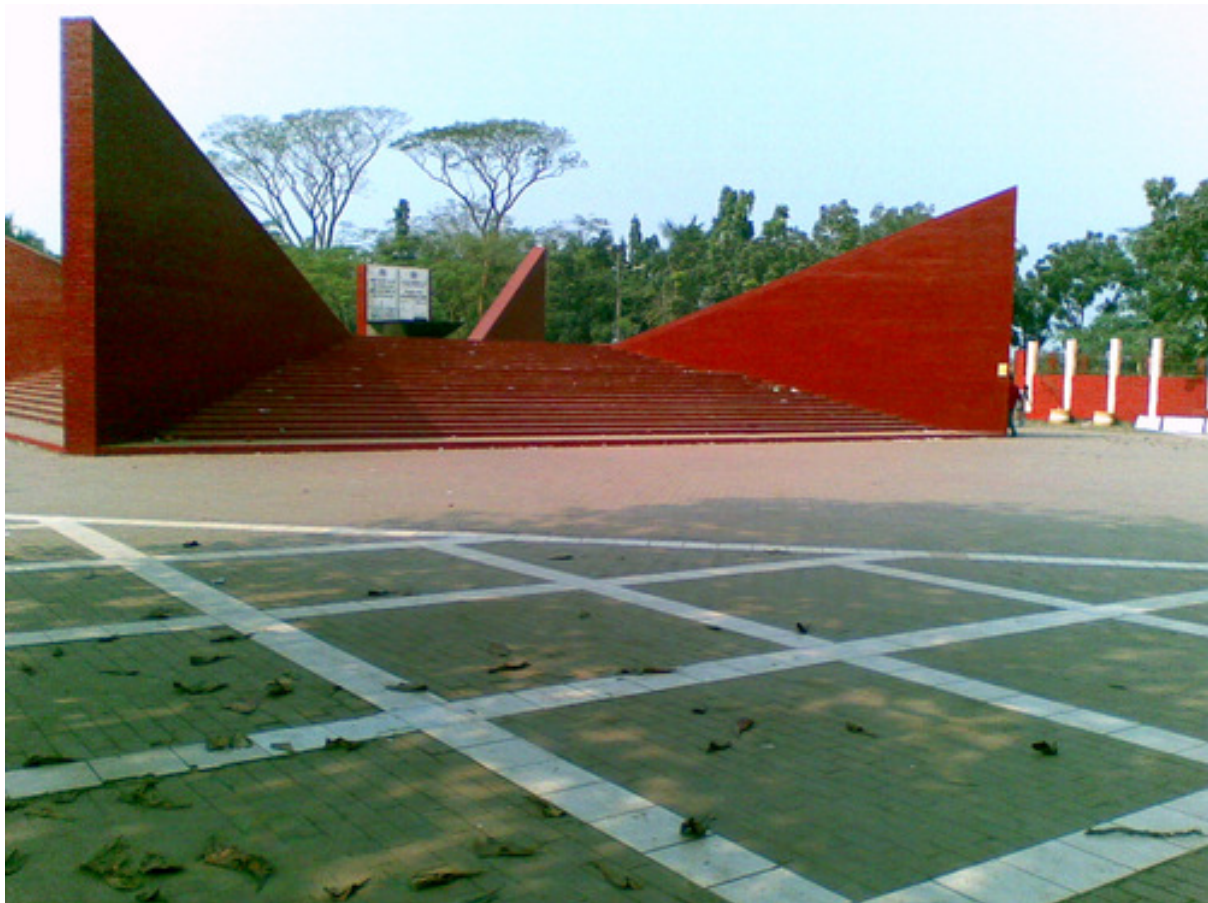
Figure 15: Public Square at Mirpur Martyred Intellectuals Memorial
