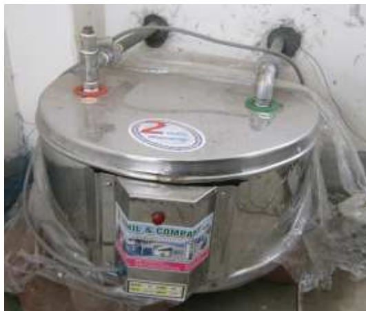
Fig.2.11: The Electric Water Heater [2].
