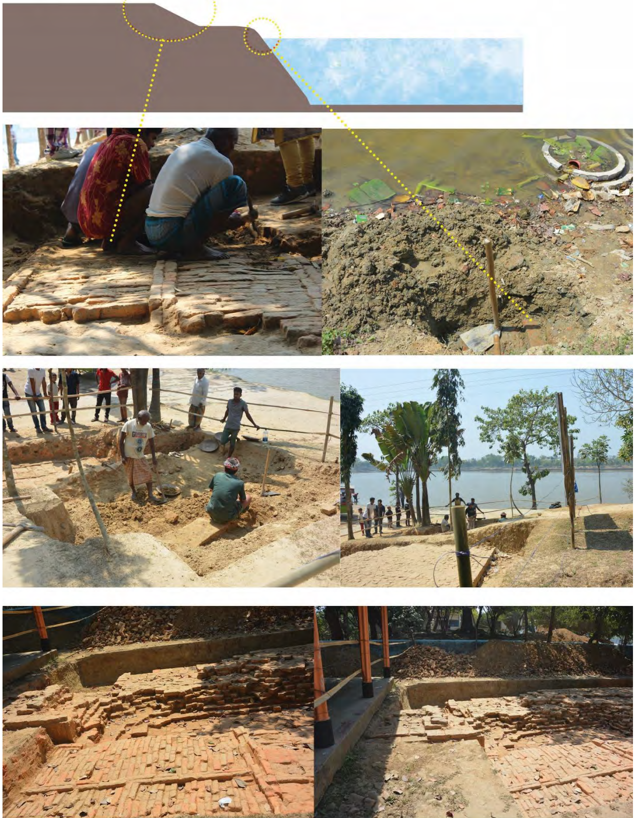
Figure 3.5.3.E x cavation. Source: Image source: Author
