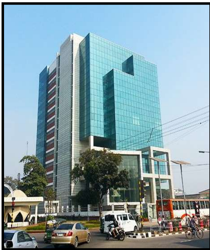
Head Office of Trust Bank Limited Shadhinota Tower, Dhaka. Gulshan 1, Dhaka
