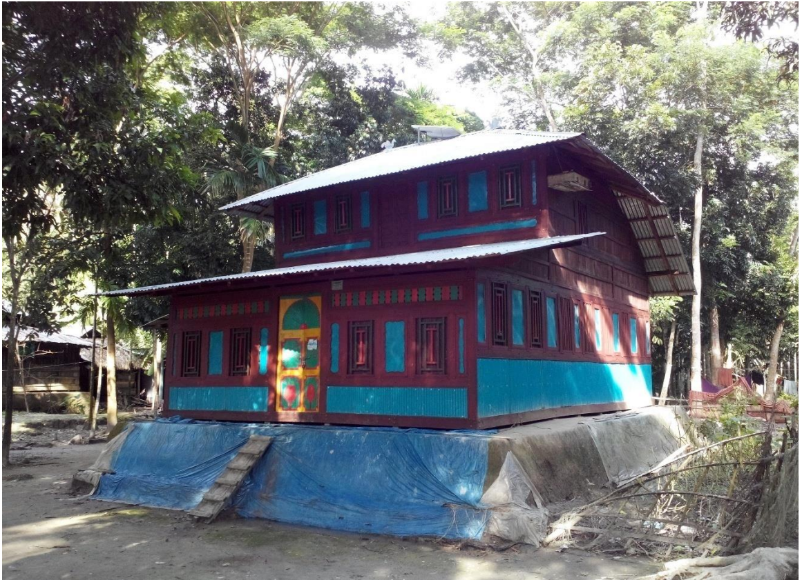
Fig 4.5: An owner built two storied house in the study area constructed after Sidrshowing fulladherence to tradition and local knowledge. Source: Author, pilot study, September 2015. The house used a jerkinhead hipped roof locally called 'takdeaghar' with enclosed pashchati in front and back. Source: Author
