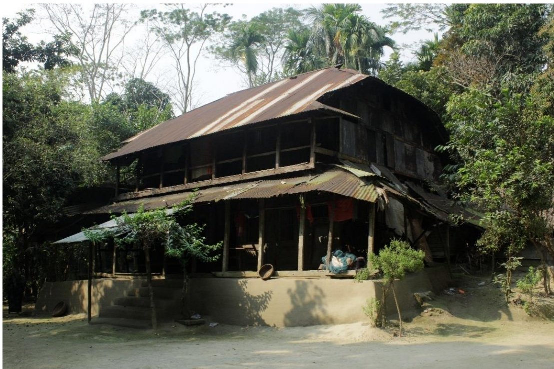
Fig 4.4b: This house, built by the current owner's father 30 years ago, survived Sidr's wrath withstanding partial damage. twelvefamily members of Hares Mollah and 10 from two neighboring houses took refuge in the upper level and survived wind and surge unharmed. He is now planning new house on the occasion of his elder son's wedding. It will be another two story wooden house of the same style with improved look
