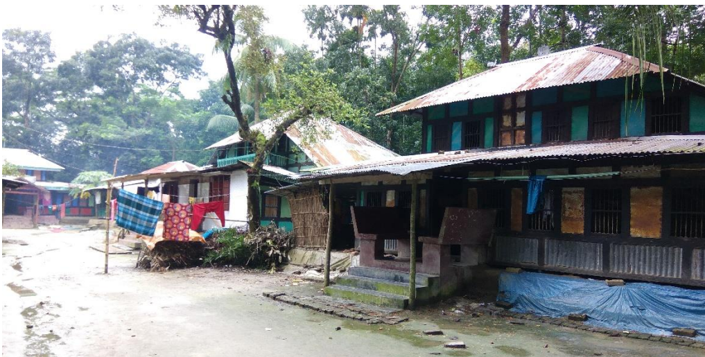
Fig 4.11a: A courtyard surrounded by traditional houses. b: A two storeid house with 'tak dea chauchal', c: a typical village settle in Barishal. Source: Author
