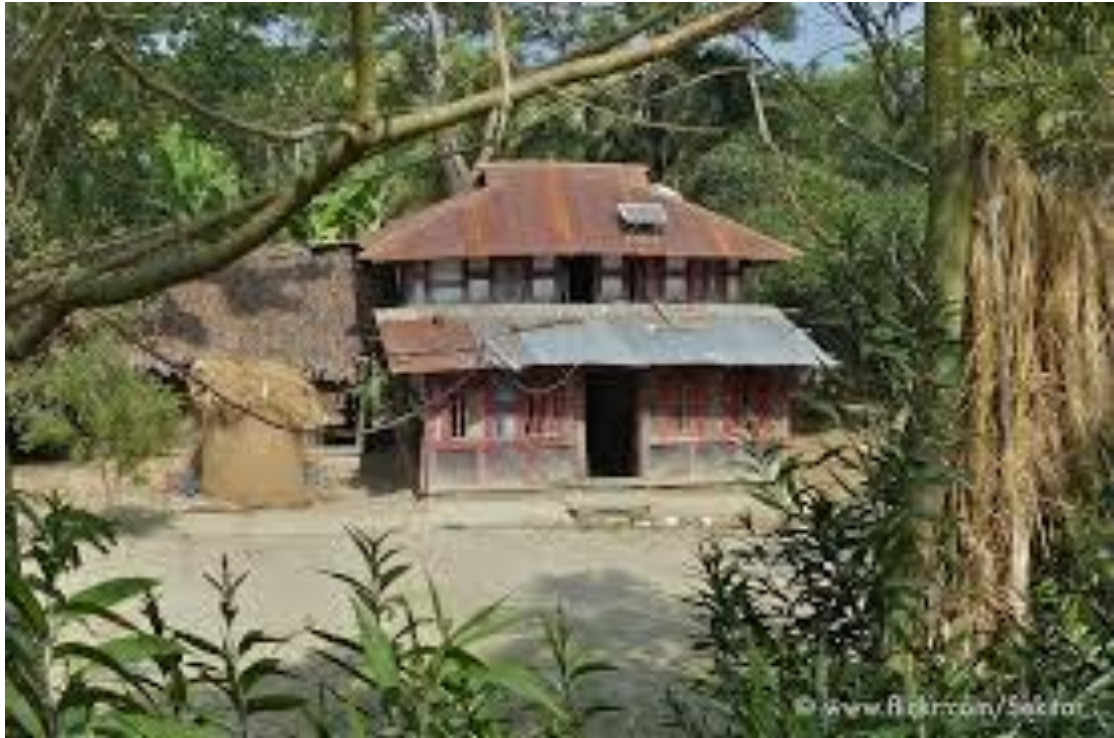
Fig 4.4a: A two storied wooden house in In Kuakata with Dutch gable Roof (chouchala) over main structure and ekchala over pashchati. Source: www.flickr.com , uploaded by sekitar
