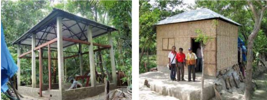
Fig. 14.13: Core shelter with additional height for mezzanine
