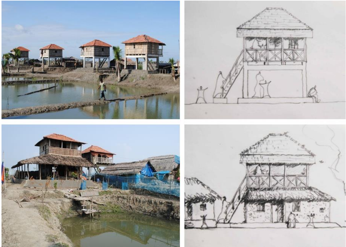
Fig 4.15: Two pictures in the left shows the settlement after completion. The elevations on the right indicates future possible adaptation by the owners, some of which are already seen in the bottom left picture where a later addition of an open paschat is visible around the resilient core structure.
