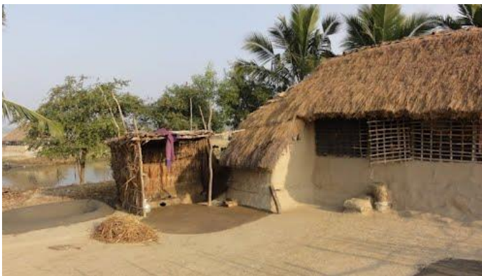
Fig 4.1 Thatched roof mud house in khulana with raised mud
