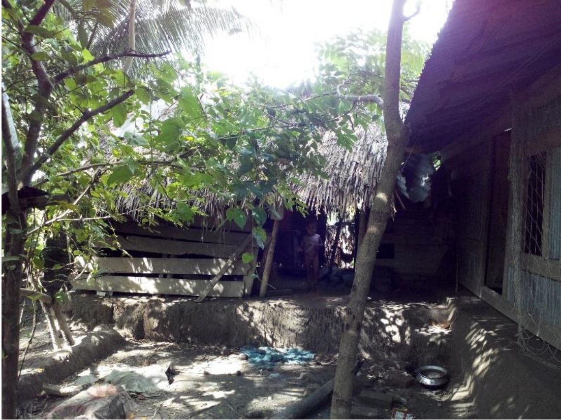
Fig 4.3: Thatch roof kitchen with bamboo posts and wooden walls in the study area. Source: author
