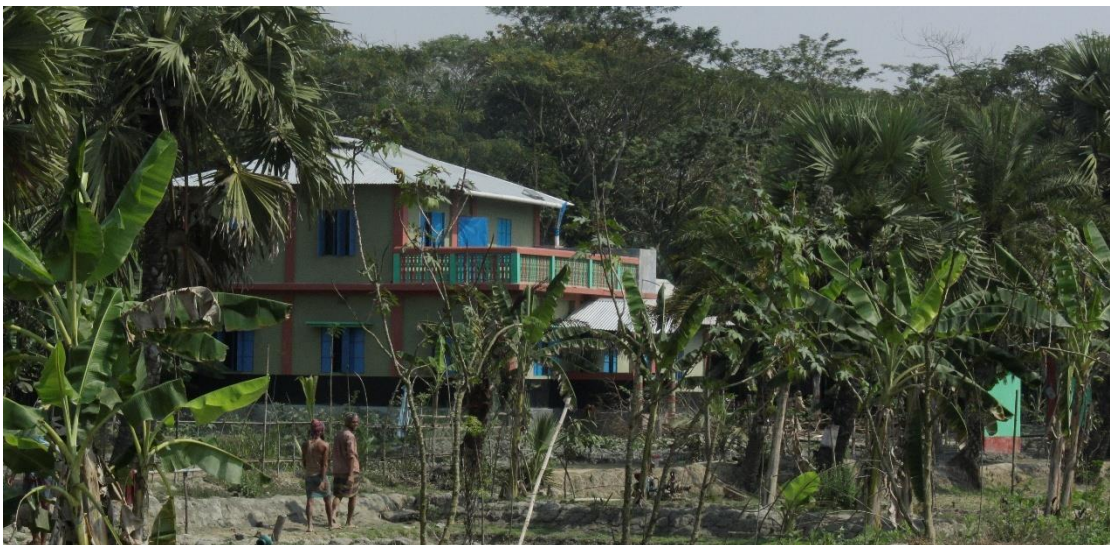
Fig 5.7: R.C.C construction following wooden precedence. (pilot study, 2015)
