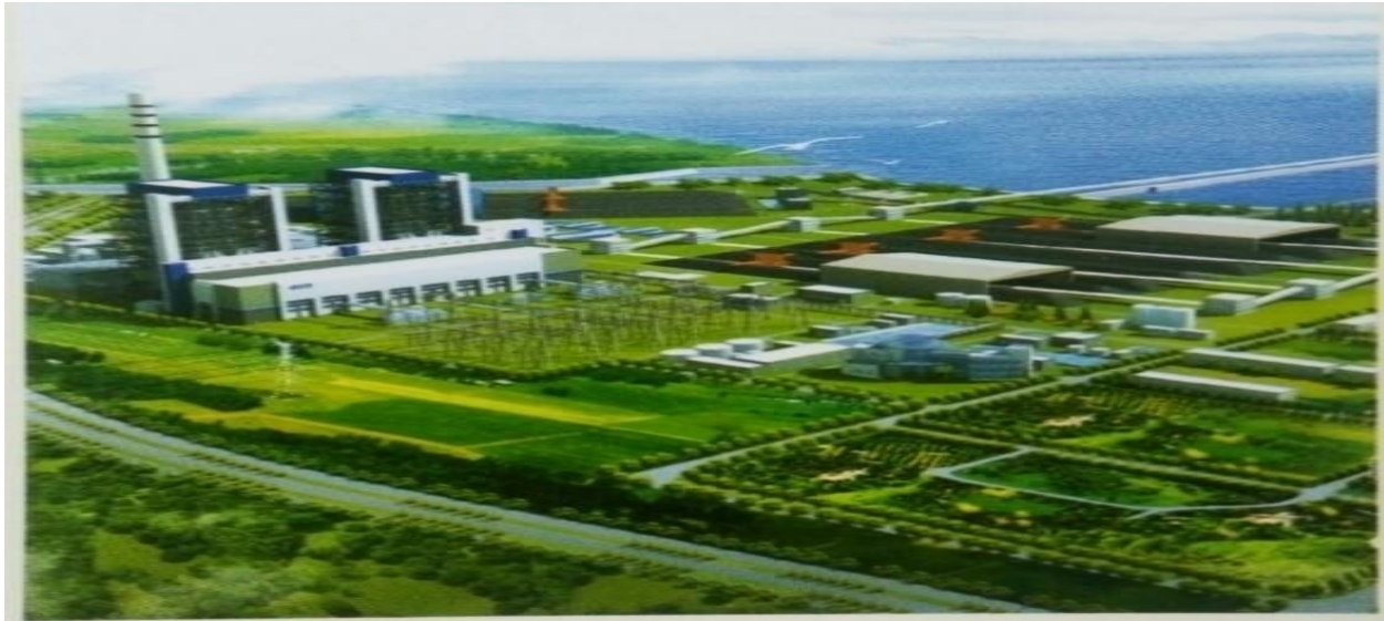
Orion Power Dhaka-2 Ltd.
