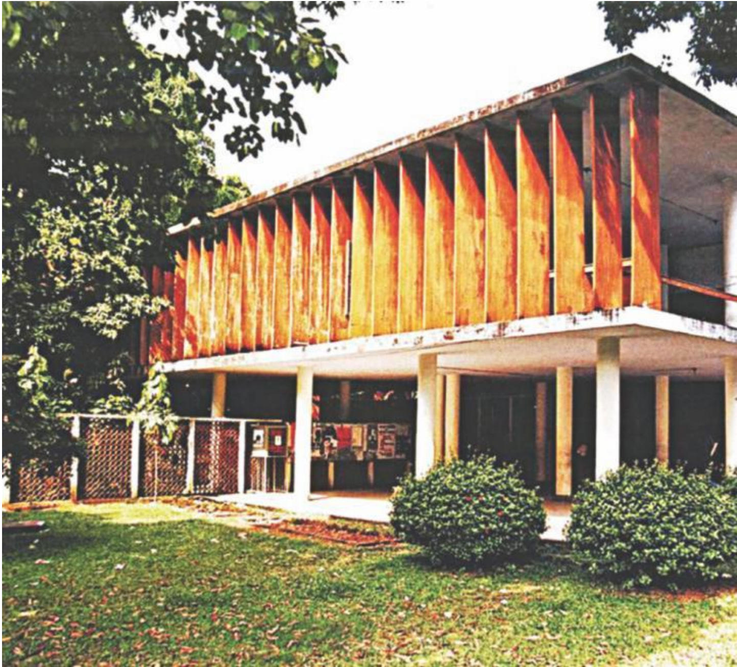
The Faculty of Fine Arts building, designed by Muzharul Islam, signalled the beginning of Bengali modernism in the architecture of the then East Pakistan. Photo: Mary Frances Dunham
