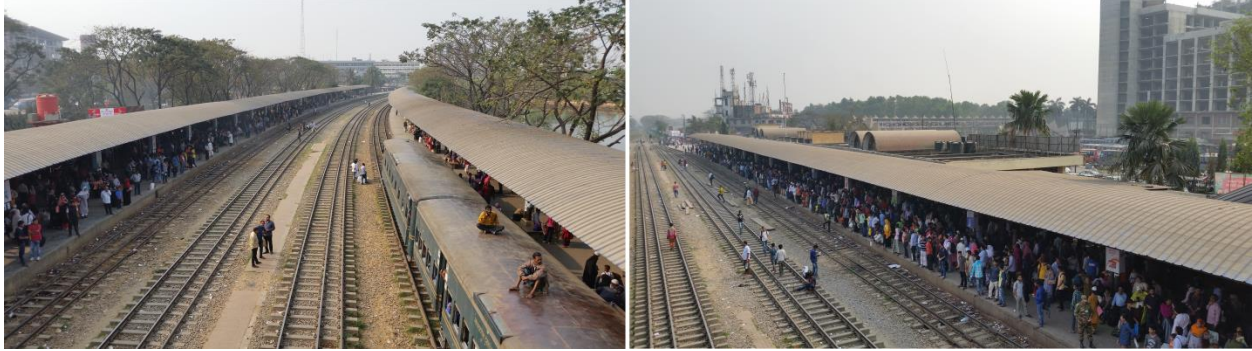
Figure 4.4.C: Existing two Platforms
