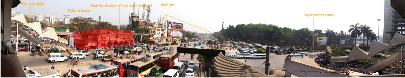
Figure 3.2.1.G: airport foot over bridge
