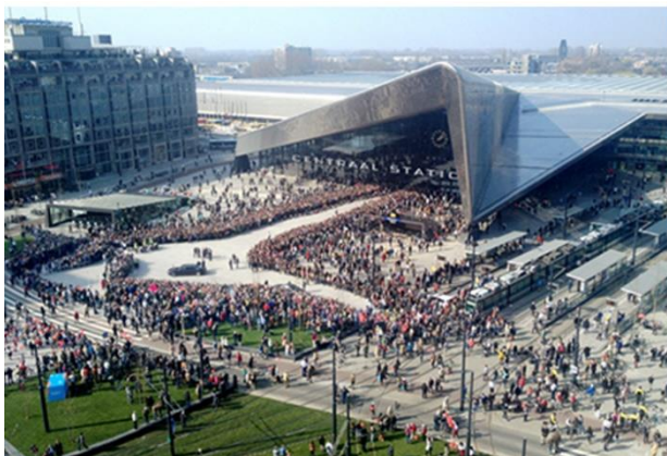
Figure 5.1.2 C: South side grand entry
