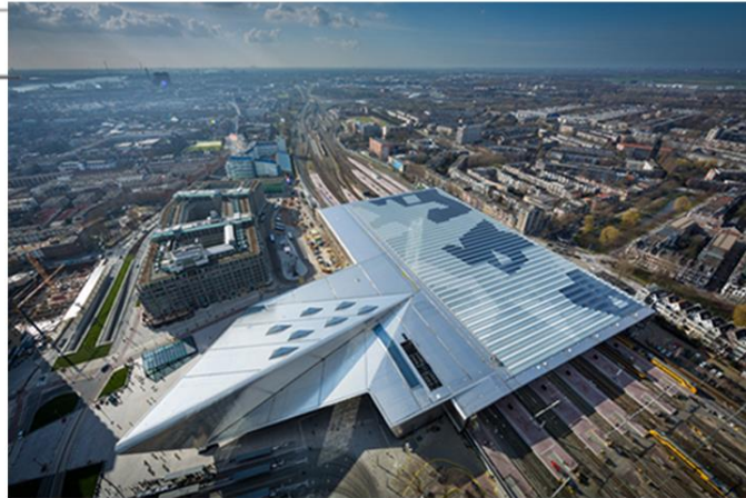
Figure 5.1.2 A: Bird view of station
