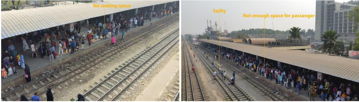
Figure3.3.D: platform of airport rail station
