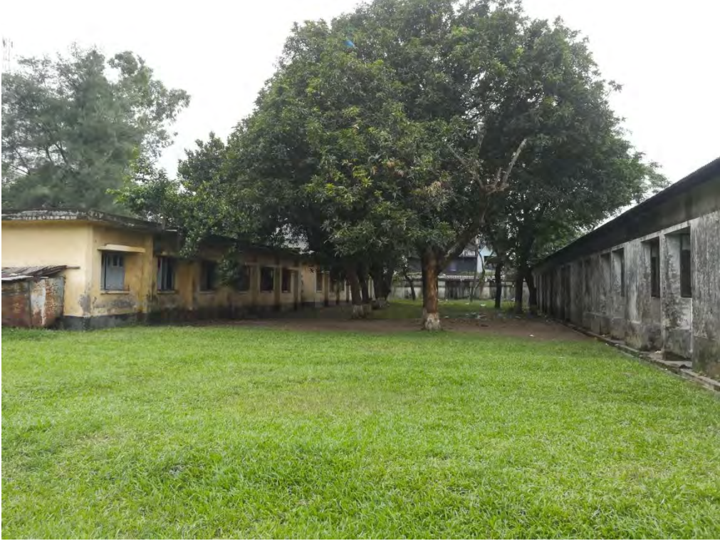
Fig 21: Inside of the site area
