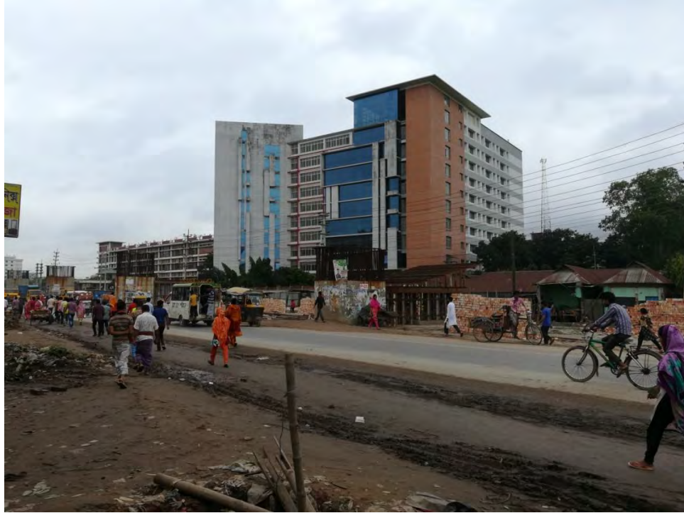
Fig 19: view from the road side
