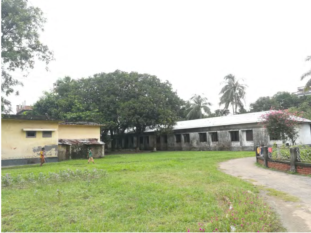
Fig 23: Inside of the site area
