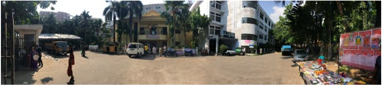
Figure: North side of the site
