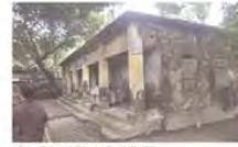
ABANDON ADMIN BUILDING
