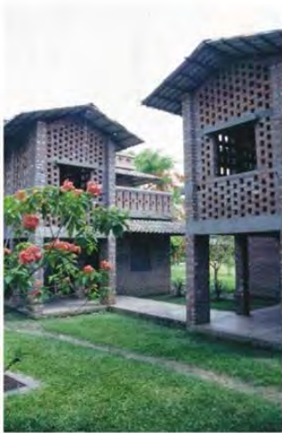
3. Trainee Hostel Stairs
