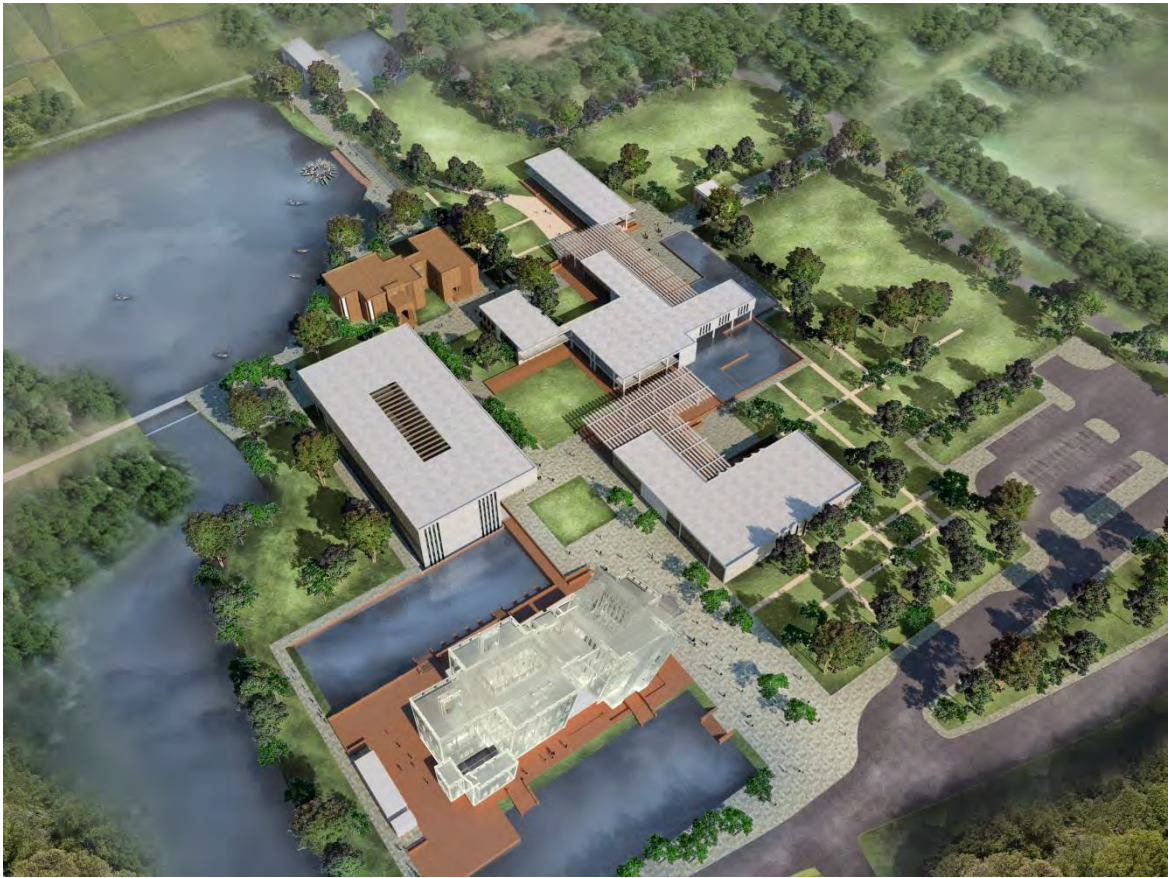
Figure 54: Aerial view of the complex
