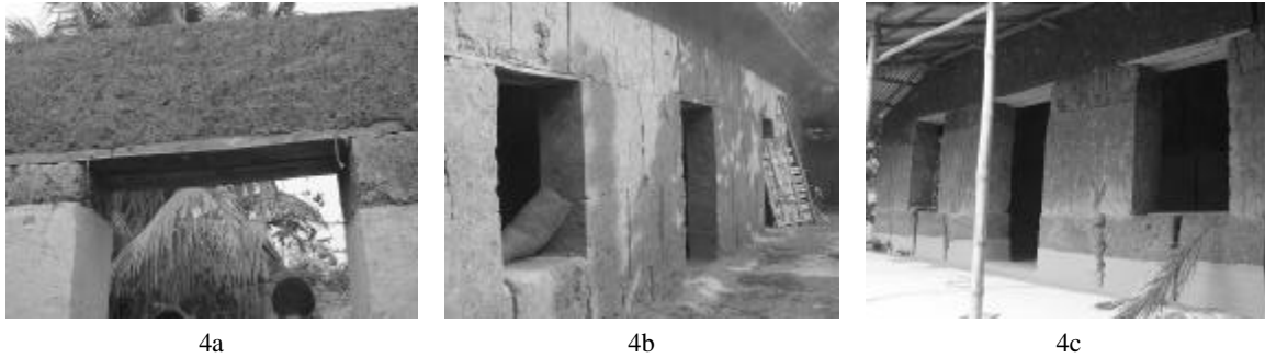
Figure 4: Wood planks are used to support load over openings
