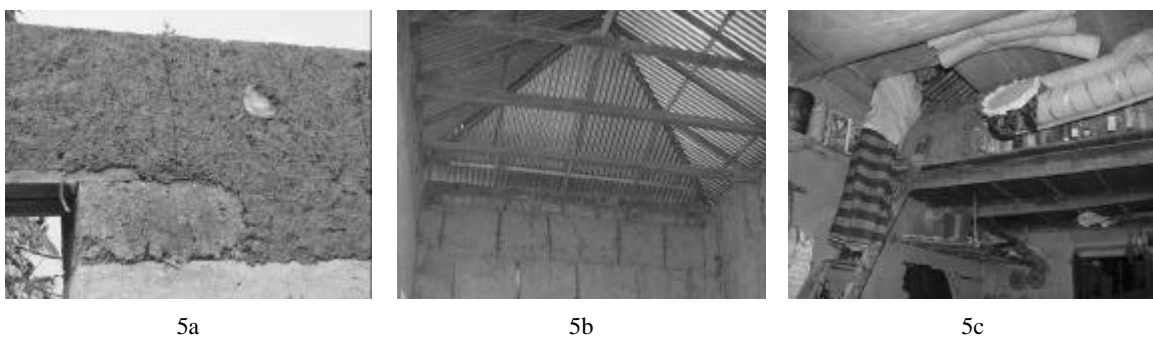
Figure 5: Wood beams made of Palm trunk and upper storage
