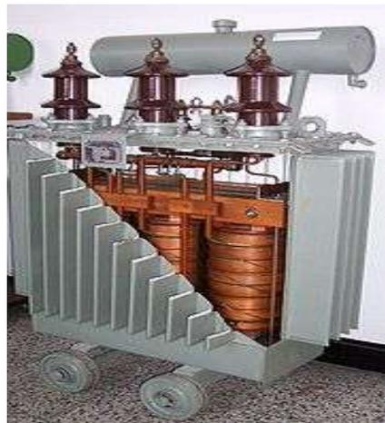
Cut-away view of three-phase oil-cooled transformer. The oil reservoir is visible at the top. Radiative fins aid the dissipation of heat.
