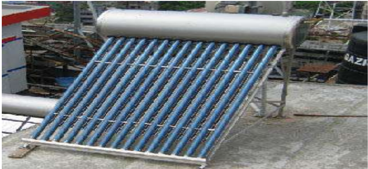
Fig2:150 liters tank with directly connected water-in-glass evacuated tube collectors
